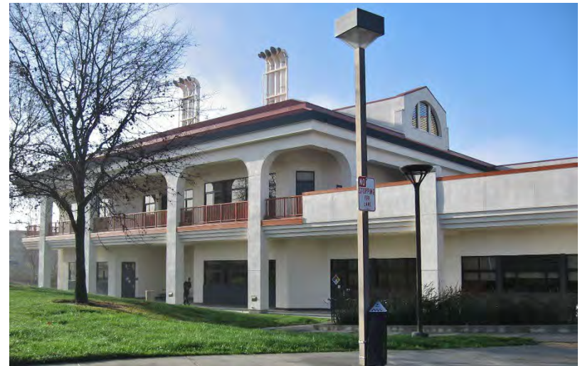
1997 Science & Tech classroom Building 1800 renovated in 2012
