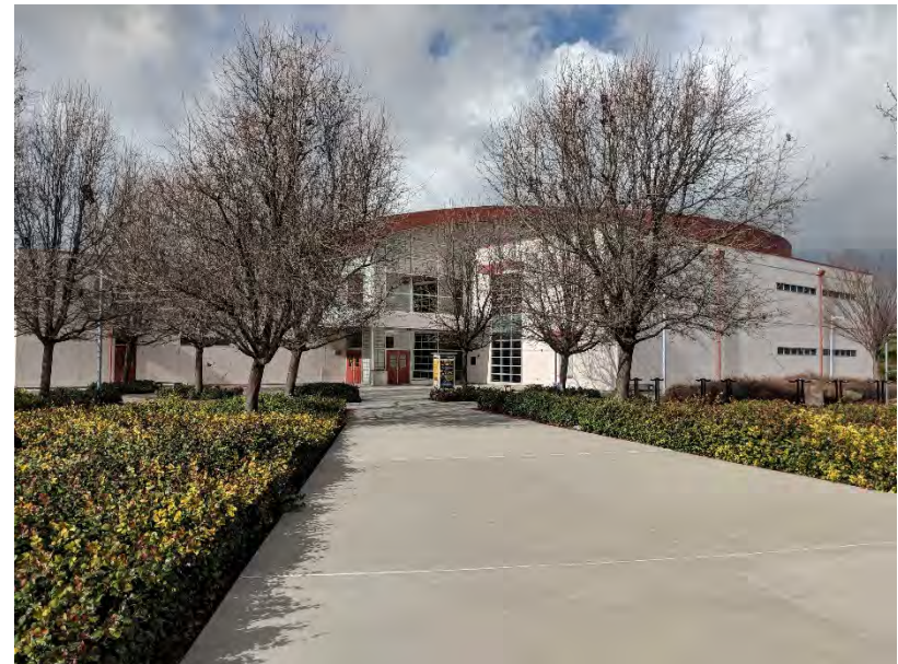
Las Positas Building 2500 P.E. Complex
