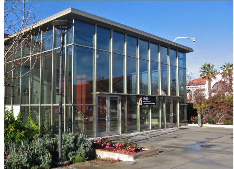
Student Service & Administration Building (B1600)
