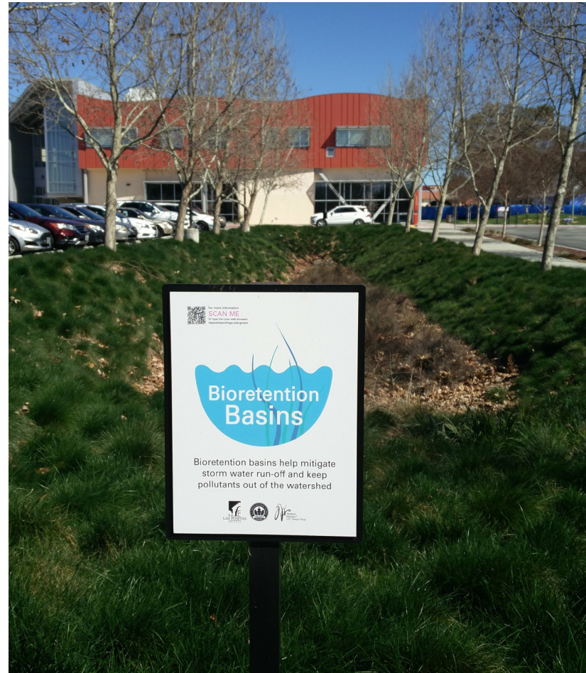
Pretreating stormwater water on site helps improve water quality.
