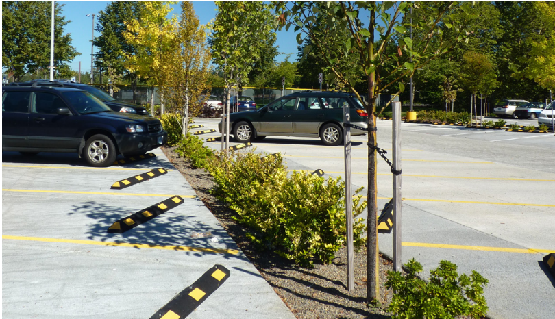
Parking lots can be retrofitted with planting areas to reduce heat islands
