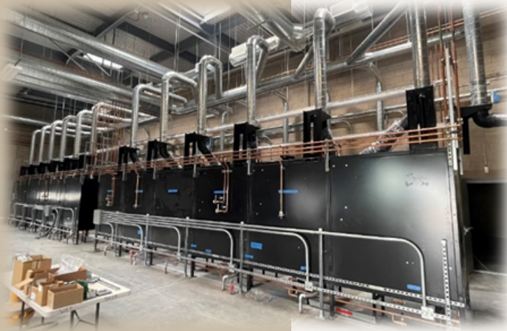
Public Safety Complex / Advance Manufacturing and Transportation
