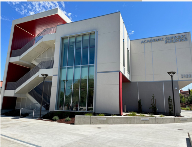
B2100 New Academic Support & Office Building
